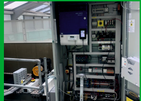
Lift Controller containing Ziehl Abegg VF Inverter Drive and Kollmorgen MPK 411 processor
