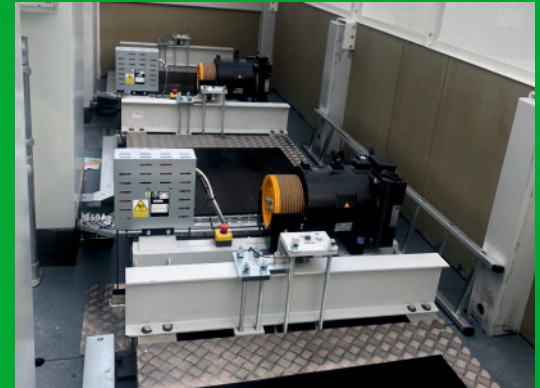
Above area now complete with the newly installed machines, support steels and over-speed governors*. Steel chequer plate was fitted between the supports.
