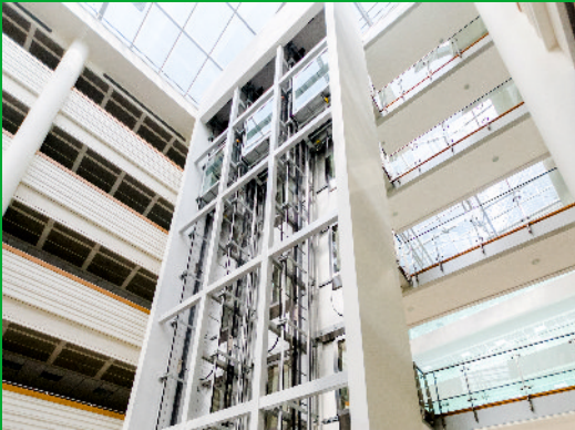
Lift installations completed and lift shaft structures cleaned and re-decorated.
