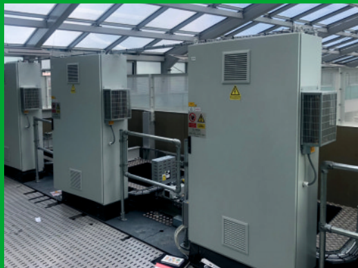
Three free standing lift controllers.
