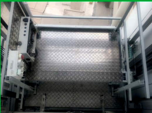
Steel chequer plate was also installed across the lift car top. This increases safety by reducing tripping hazards but also for aesthetic purposes. Lift car top handrail raised and strengthened.
